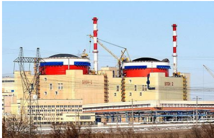
Russia, Rostov NPP Unit 2 - 1000 MW
