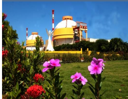
India, Kudankulam NPP Unit 1 - 1000 MW
