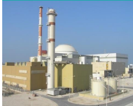
Iran, Buser NPP Unit 1 - 1000 MW
