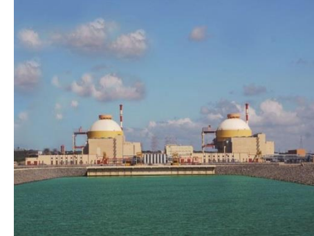
India, Kudankulam NPP Unit 2 - 1000 MW
