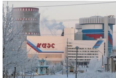
Russia, Kalinin NPP Unit 4 - 1000 MW
