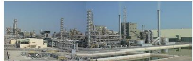
Ammonia / Urea Plant (Oman)
